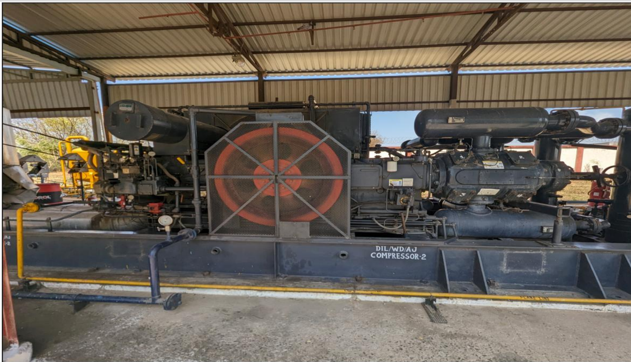
Exhibit 19: Gas Compression Equipment ( Gas Compressor)
