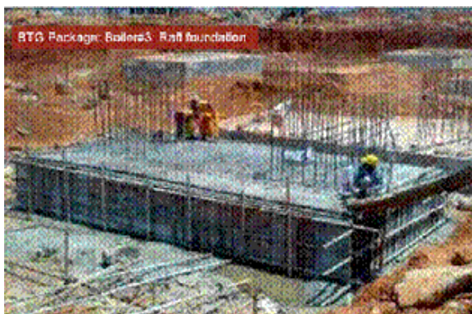
PROGRESS AT THE UTKAL PROJECT
