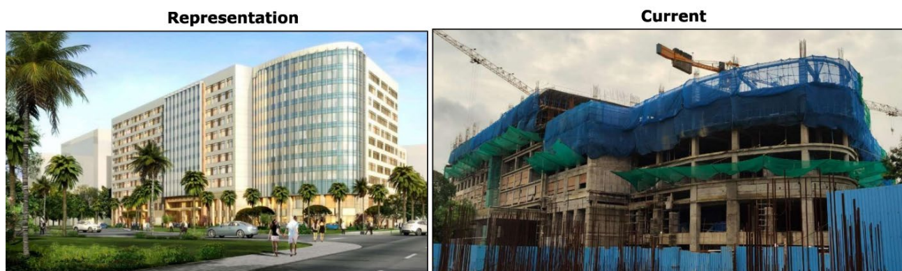
Fig 7 – Lemon Tree is set to open its largest hotel, Aurika (669 rooms), Mumbai (MIAL) by end-CY23
